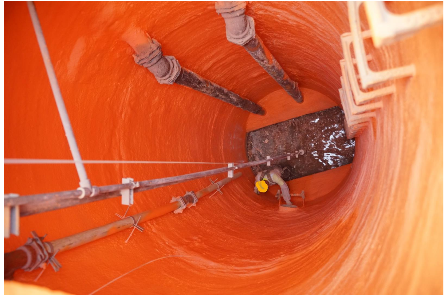
8' Diameter 34' Deep Sanitary Sewer Pump Station
