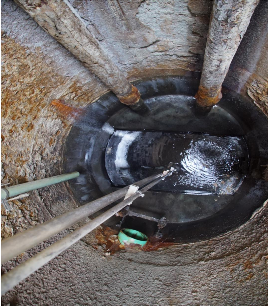
8' Diameter 34' Deep Sanitary Sewer Pump Station
