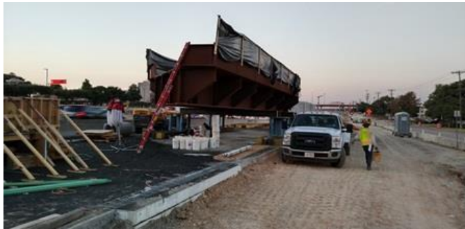
“south-bound” deck location
